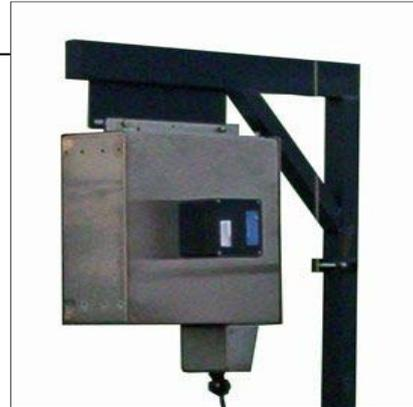
The Signaline auto Cable collector is fixed above the floating roof tank with the cable retracting from the bottom. This allows the cable to stretch and retract as the tank raises and lowers. Above shows the fixings of the cable reeler. Below is a diagram outlining the system.
